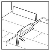
Fix skirting boards or scotia using quality construction adhesive and/or brads or small diameter nails. It is important to never attach or glue the skirting board or scotia trims to the floor. This method allows the floor to expand and contract under the
