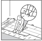
**HINT:** To obtain a clean cut, use a fine teeth, scroll cut blade when using a jigsaw or circular saw. The use of saw blades that have a higher amount of cutting teeth is also recommended to achieve a neat cut.
